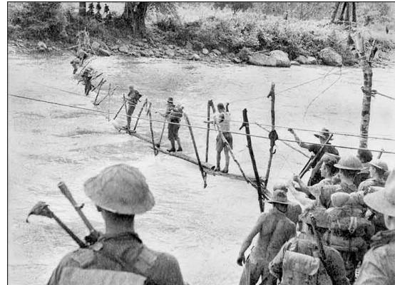
Kumusi River Bridge
